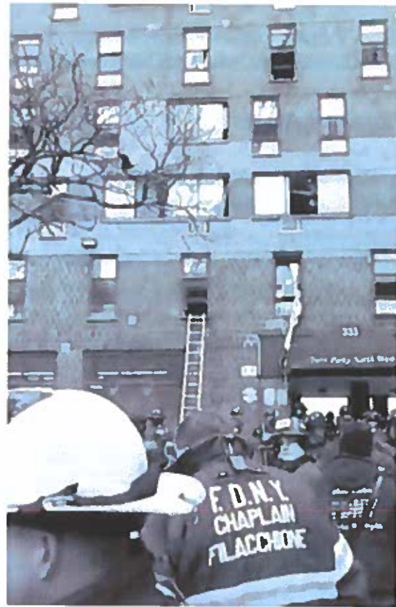
FATAL FIRE: Firefighters use ladders to access units in a 19-story apartment building that caught fire in the Bronx in New York Sunday. The fire killed 19 people, many of them children, in what officials called one of the most devastating blazes in city history. Screenshot of a video by The Washington Post
